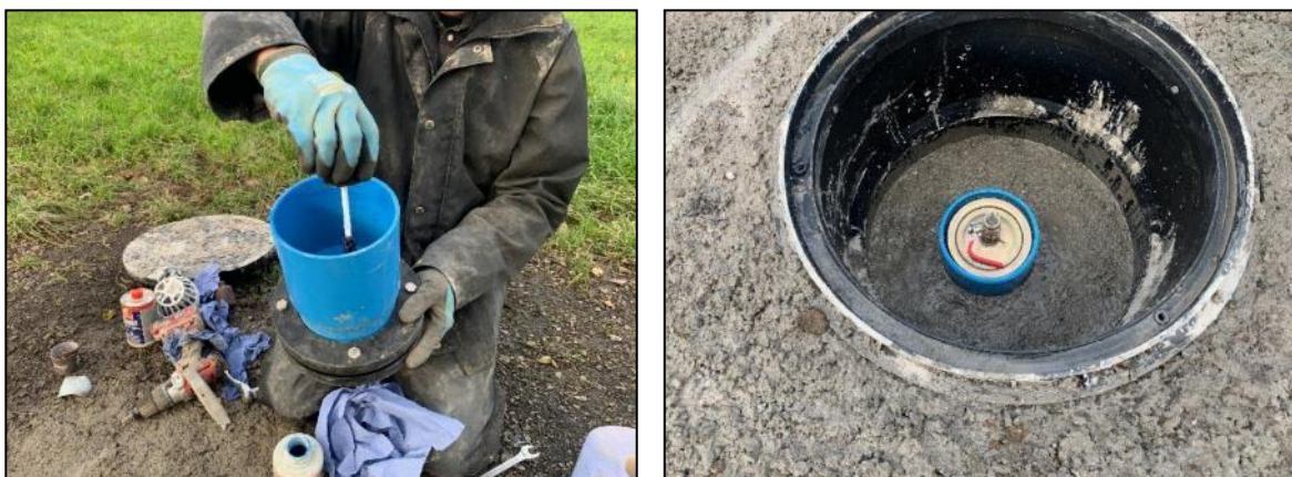
Figure 56 (Left) Applying glue to a uPVC top cap. (Right) Temporary plug to glue on top cap.
