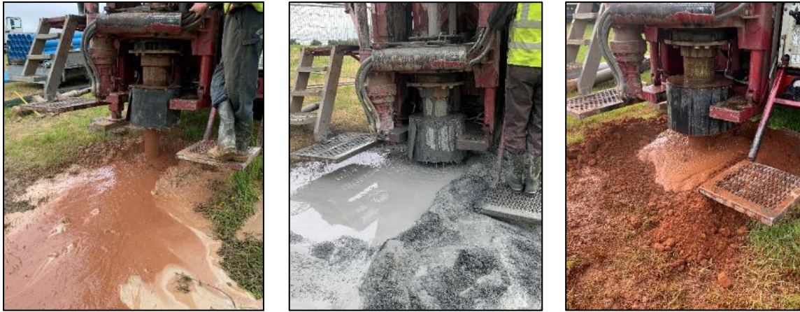
Figure 52 Drilling returns from boreholes 1, 2 and 3 (left to right)
