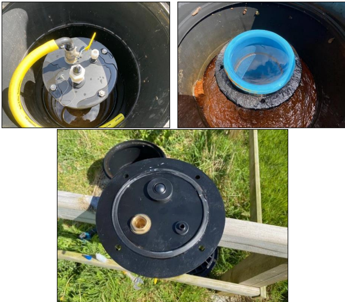
Figure 57 (Left) Modified nylon artesian well top flange plate with sample tap, air valve and pressure logger bulkhead fitting. (Right) Open borehole showing nylon flange ring below uPVC edge. (Bottom) Underside of nylon top flange plate showing the all important O ring glued in place.
