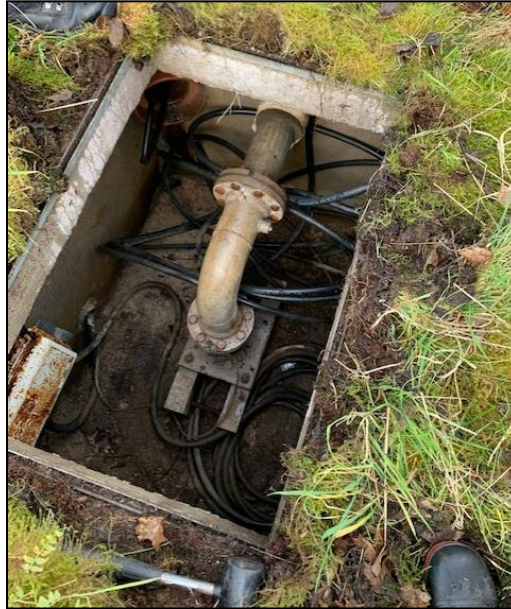
Figure 3: Inspecting a former production borehole
