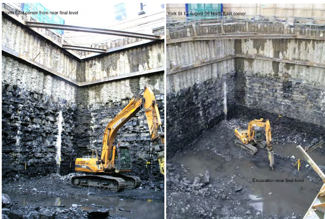
Figure 5 – York St. Basement Excavation (McNamara Construction)
