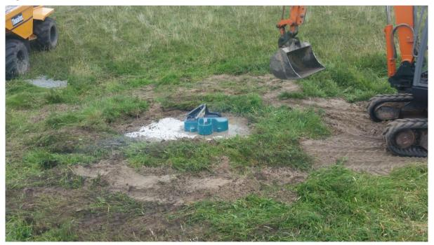
Figure 66: Pasture pump – one of 4 across the site, utilising groundwater for cattle. Access Umbra burn closed.
