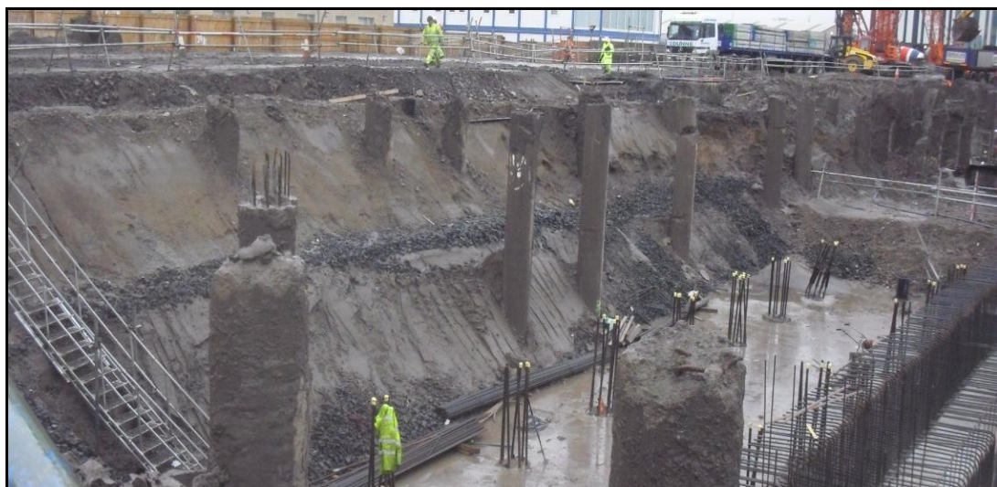
Figure 16. Construction of stable slopes with vacuum wells & passive angular stone drains
