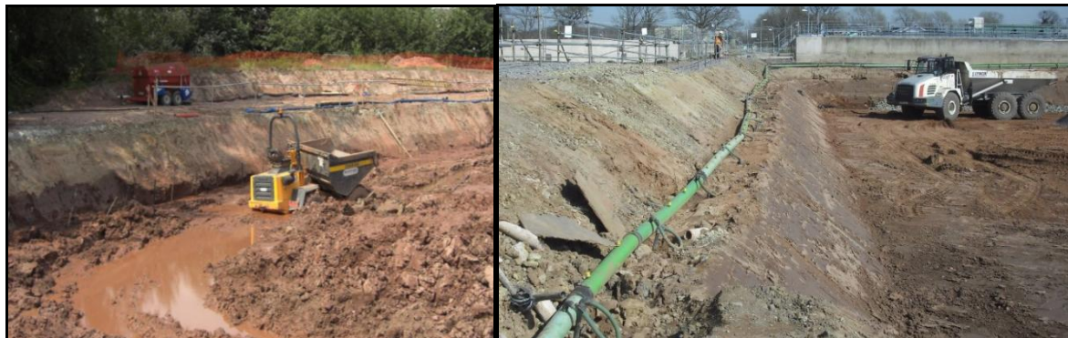
Figures 6 & 7. Sump pumping of groundwater versus using a wellpointing operation
