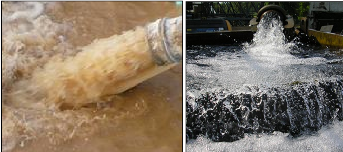
Figures 8 & 9. Discharge of water from sump pumping versus discharge from wellpointing Changes effective resulting from the lowering of the water-table
