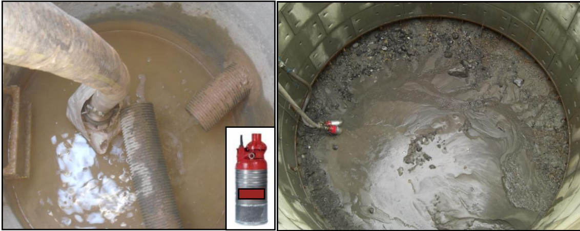
Figures 4 & 5. Traditional sump pumping from shafts
