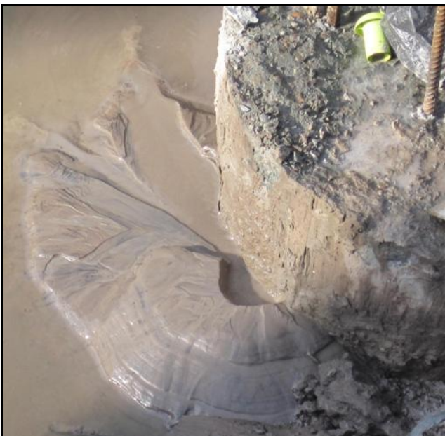
Figures 13 & 14. Seepage alongside a curing concrete pile from an artesian stratum.
