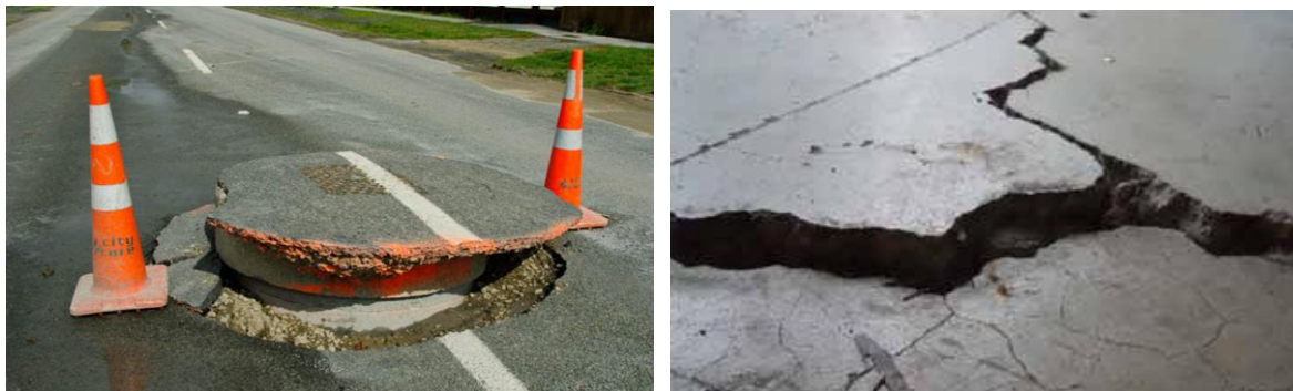
Figures 17 & 18. Examples of structural uplift, including cracking of a concrete slab.
