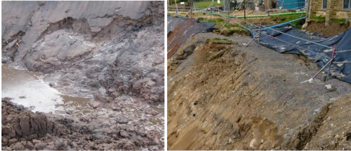
Figures 29 & 30. Soil deformation as a consequence of slope embankment failure.
