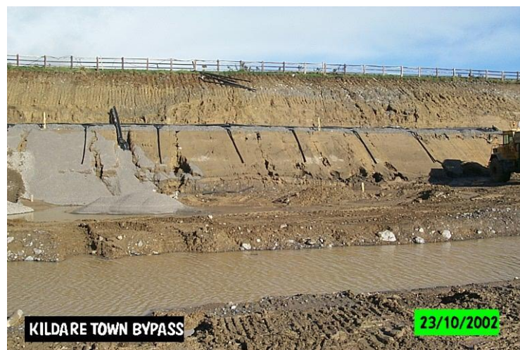
Figure 4: Large scale sump pumping.
