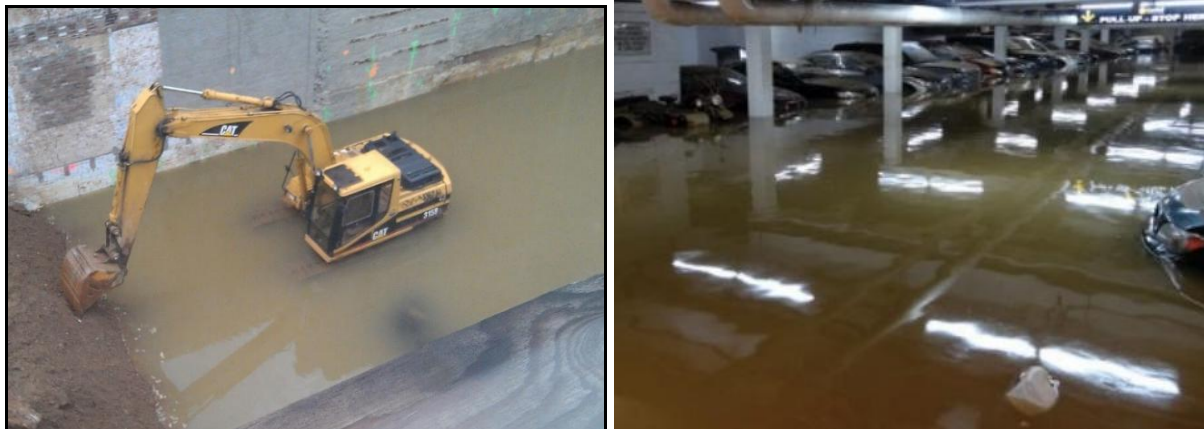
Figures 2 & 3. A construction site and parking basement with inundation from groundwater
