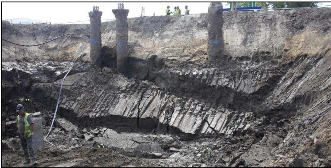
Figure 15. Progressive slope failure caused by a saturated soil layer at the toe
