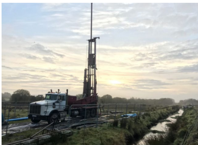
Figure 3: Groundwater monitoring borehole drilling
