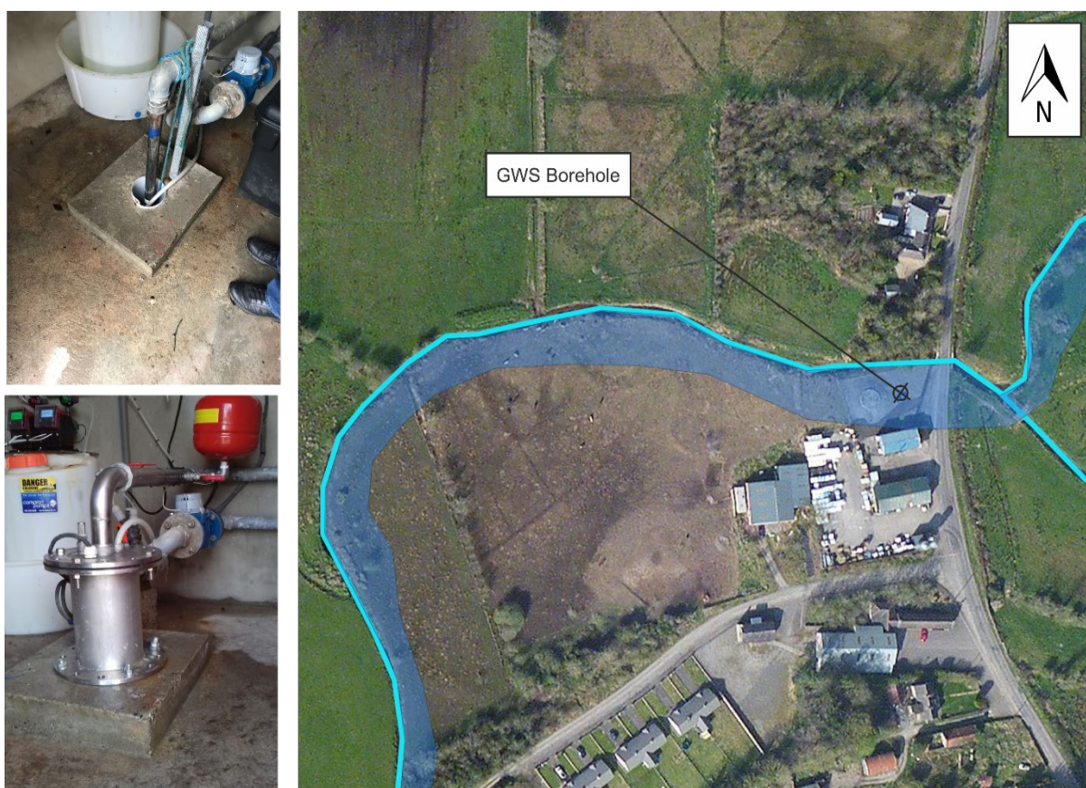
Figure 5a (Top Left). Borehole at Ballyallen GWS, Co. Carlow. Figure 5b (Bottom Left). Borehole at Ballyallen GWS, post well head improvement works.
