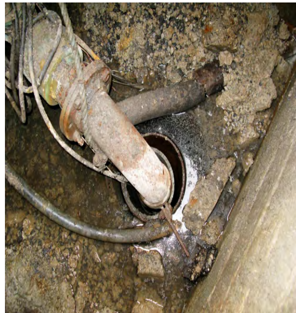
Figure 2.2 is the wellhead above an old borehole
