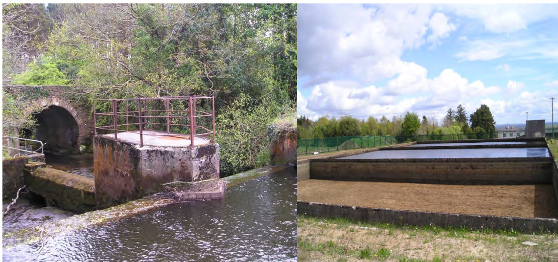
Figure 2.1 The Catholes showing the intake on the left and the slow sand filters on the right
