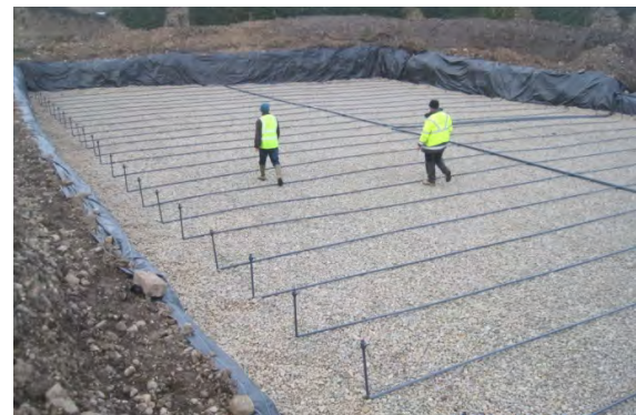
Photo 2: Feb 2014, installing the pressurised distribution pipework in one of the soil polishing filters.
