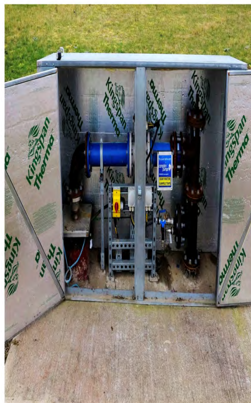
Figures 3.2 shows a modern control Kiosk mounted on top of a wellhead pad
