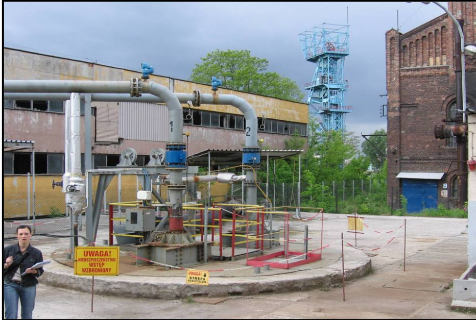
Figure 1. Katowice mine shaft (with dewatering pumps) in an urban environment in Poland (photo by © David Banks).
