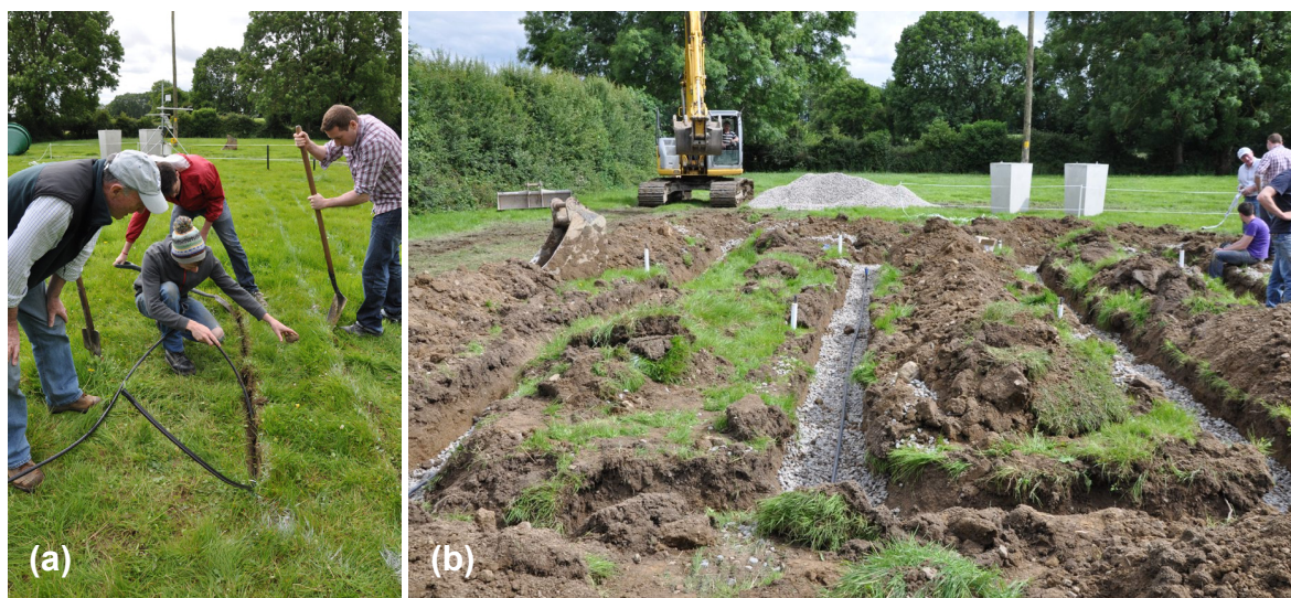
Fig. 2. (a) Installation of DD tubing, and (b) LPP system.
