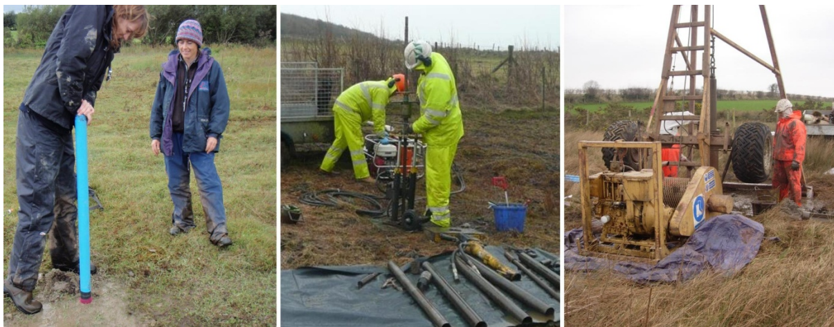
Figure 10 Left: affordable dipwells can be installed by hand to a depth of 2-3meters in unconsolidated materials (Rhoswen Leonard and Janine Guest). Middle: slightly more expensive power hand drill can install to a greater depth and through more competent materials. Right: a large percussion drill can install a borehole or piezometer into more competent material (photograph Dr Peter Jones).
